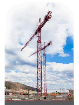
Two tower cranes, which are 300 and 360 feet tall, were installed in early 2018 as part of the construction of UPF. Having high-capacity, stationary cranes within the footprint of the buildings gives UPF the ability to reach every spot in the construction zone, making materials handling safe and efficient.
