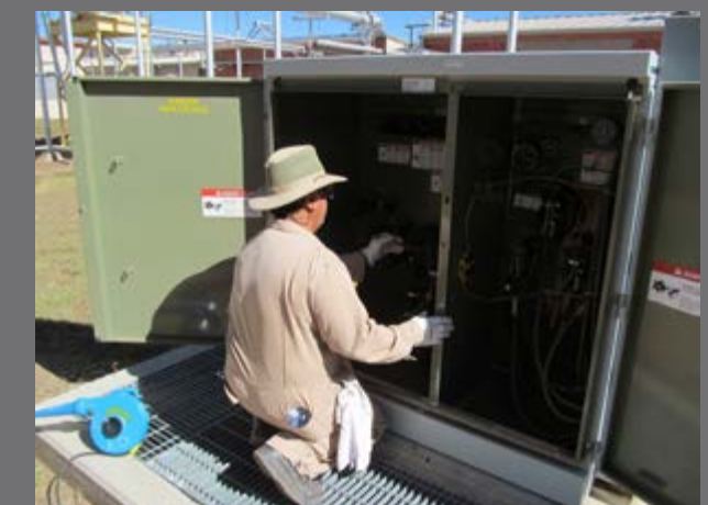
Frankie Diaz at Pantex cleans the interior of a de-energized 12,470/480-volt transformer.
